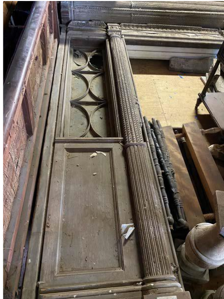
Photograph of the purported original door frame and surround, featuring highly decorative beaded and fluted pilasters and sidelights with wood panel. [National Trust for Historic Preservation, 2020]
