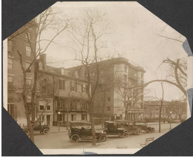
The Cameron House (the old Benjamin Ogle Tayloe House) on Lafayette Square in 1916. Next door was the Belasco Theatre, which caused Cameron to leave the house because of the noise it generated. Image: Wikipedia.
