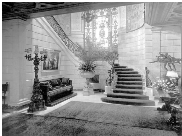
Staircase of Lyndhurst.
