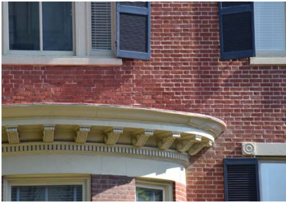
Fig. 25 [Top Left] Bent section of cornice at entrance bay on right. [BBB, 2024]
