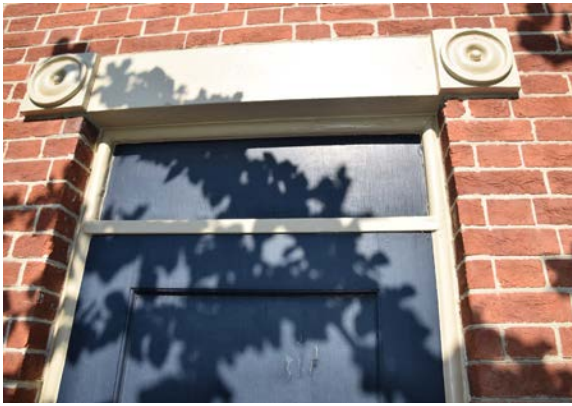
Fig. 41 [Top Left] Deteriorated finish at wood door on east façade. [BBB, 2024]
