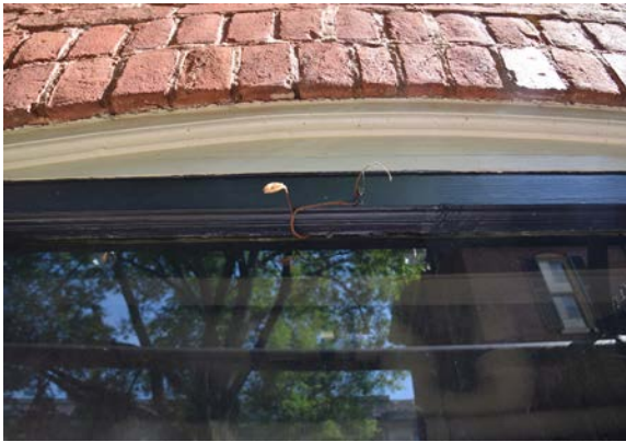
Fig. 43 [Center Left] Plant growing out of transom window above western door on south façade of the Carriage House. [BBB, 2024]
