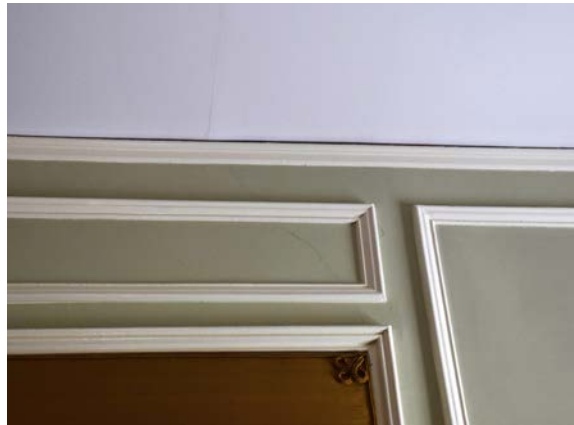
Fig. 58 [Right] Hairline crack in plaster ceiling and wall panel in North Parlor. [BBB, 2024]
