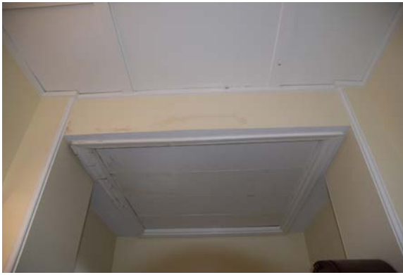
Fig. 61 [Top Left] Staining at ceiling finishes on third floor. [BBB, 2024]
