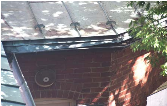
Fig. 27 [Left] Displaced and bent copper flashing at the copper gutter on the Carriage House. [BBB, 2024]
