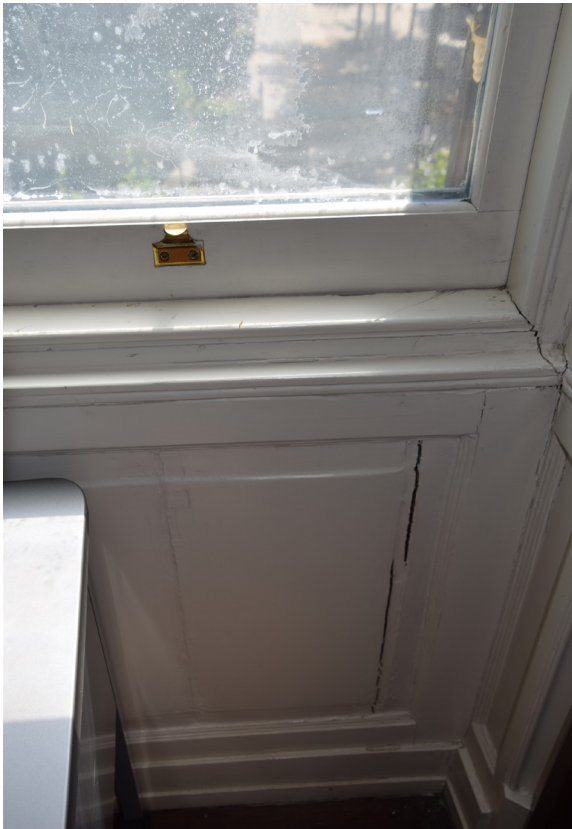
Fig. 73 [Lower Left] Split in panel at window apron on third floor. [BBB, 2024]
