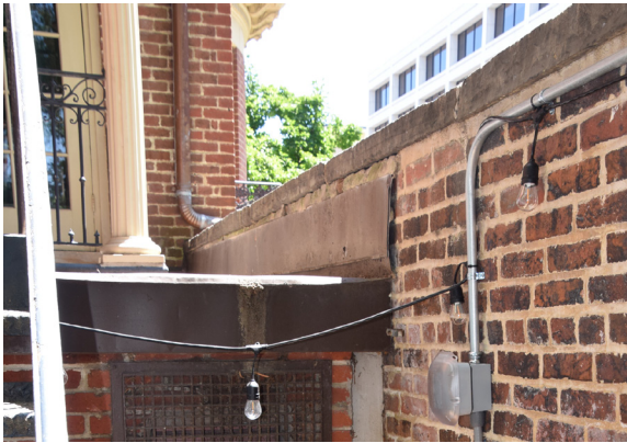
Fig. 12 [Left] Failing mortar at coping stone of garden wall. [BBB, 2024]
