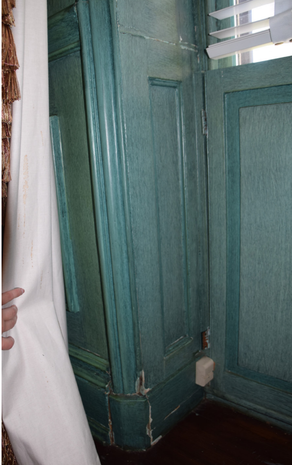
Fig. 54 [Lower Left] Joint separation and deteriorated finish at window jambs and baseboard in Garden Room. [BBB, 2024]
