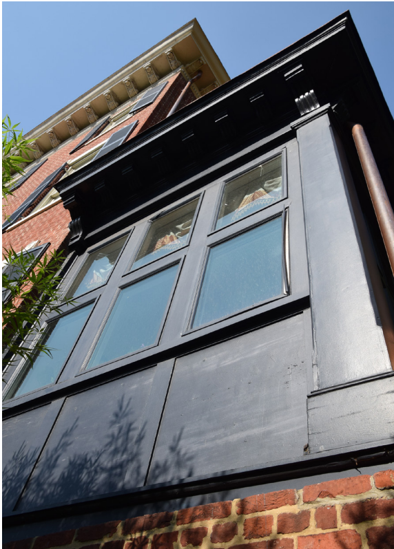
Fig. 45 [Lower Left] North porch showing minor deterioration of finish and missing/ detached window trim. [BBB, 2024]
