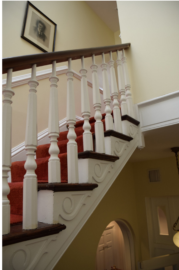
Fig. 67 [Top Left] Stair conditions ascending to fourth floor. Stairs slope slightly away from wall and should be monitored. [BBB, 2024]
