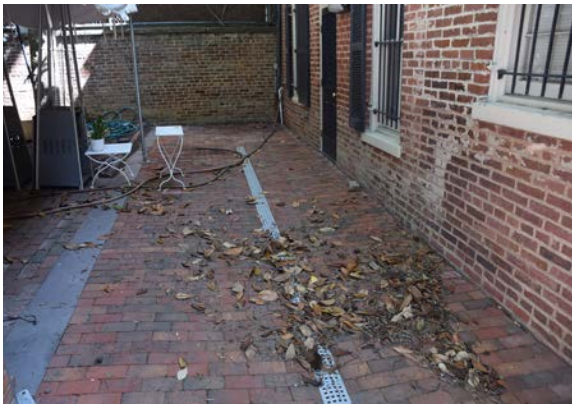
Fig. 14 [Left] Newly installed drain along west side of the Car- riage House. [BBB, 2024]
