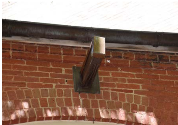
Fig. 50 [Lower Left] Separating joint at frame of east balcony on south façade. [BBB, 2024]
