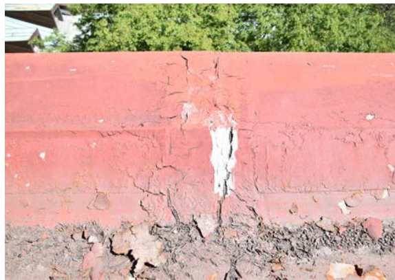
Fig. 19 [Left] Detail of roof showing deterioration of paint and flattened seams. [BBB, 2024]
