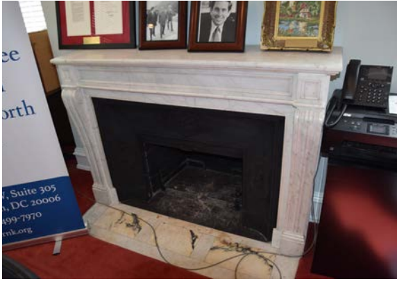
Fig. 71 [Top Left] Settling of fireplace in northeast office on third floor. [BBB, 2024]
