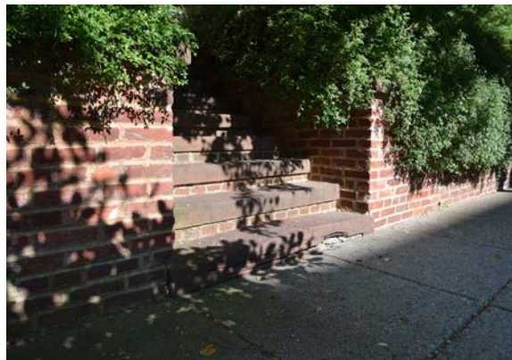
Fig. 5 [Left] Erosion and existing patches to be monitored at front steps. [BBB, 2024]
