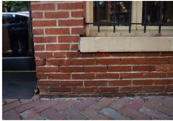
Fig. 33 [Top Left] Open joints at pressed brick at front entrance bay. [BBB, 2024]
