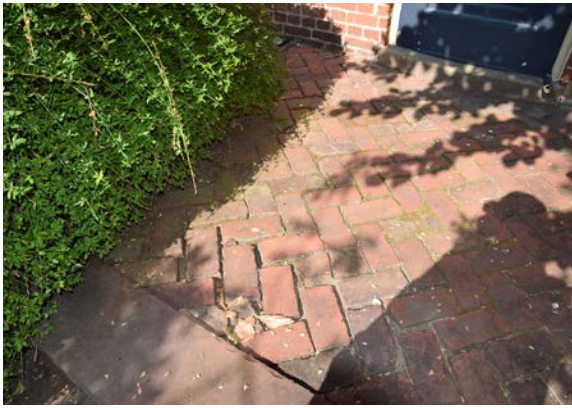
Fig. 10 [Top Left] Loose bricks at landing of east stair. [BBB, 2024]
