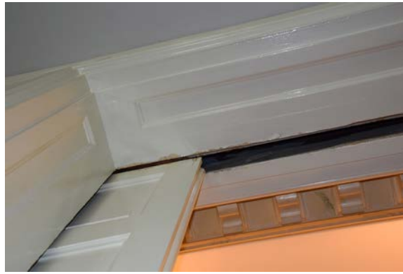
Fig. 56 [Top Left] Hairline cracks at corners of Gallery pilasters. [BBB, 2024]
