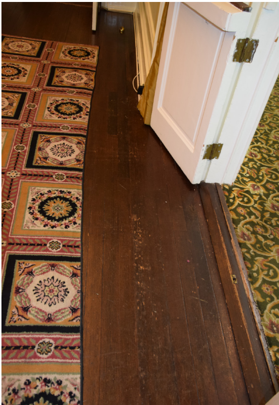
Fig. 65 [Bottom Left] Worn finish at wood floors in Dining Room. [BBB, 2024]
