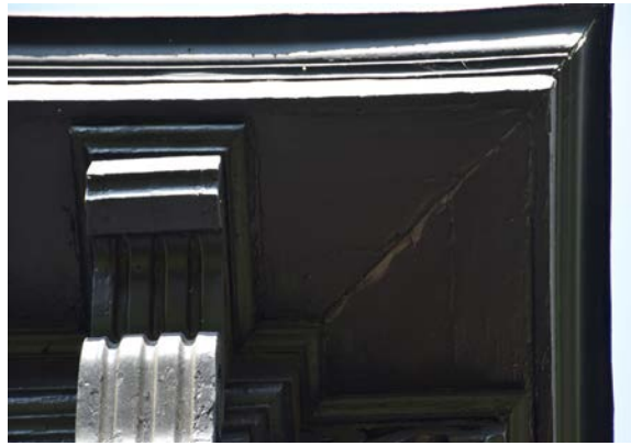
Fig. 46 [Top Left] Exposed wood beam at east façade of north porch, deteriorated finish at wood elements above. [BBB, 2024]
