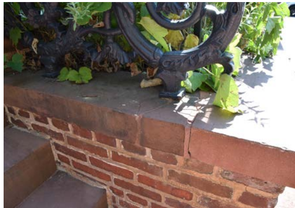
Fig. 3 [Left] Open joint at coping stone at retaining wall. [BBB, 2024]
