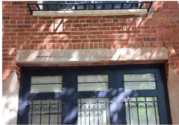
Fig. 35 [Left] Sandstone at front bay exhibits ero- sion and should be monitored. [BBB, 2024]
