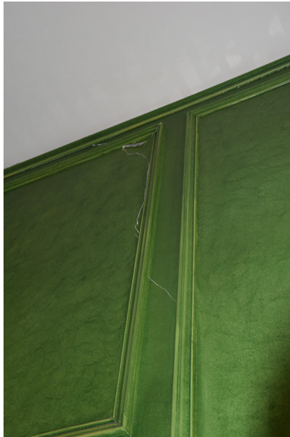
Fig. 59 [Lower Left] Separation at crown molding and vertical crack at northwest corner of South Parlor. [BBB, 2024]
