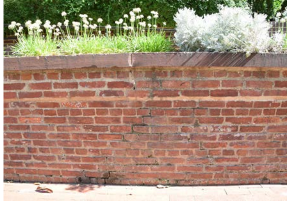
Fig. 1 [Top Left] Retaining wall on south façade is leaning from hydrostatic pressure. Continue to monitor. [BBB, 2024]
