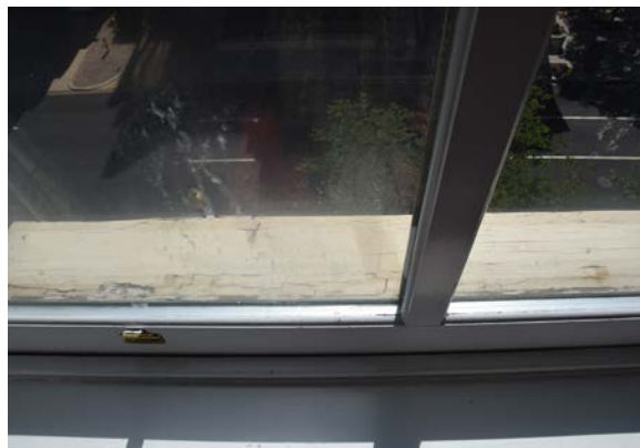
Fig. 39 [Lower Left] Deteriorated finish and minor checking at the wood window sill and lintel on the east façade. [BBB, 2024]
