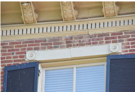
Fig. 31 [Lower Left] Fracture crack at lintel and step crack above on south façade. [BBB, 2024]
