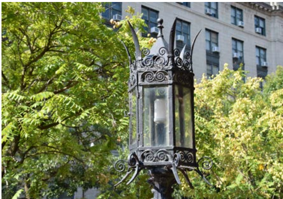
Fig. 16 [Lower Left] Wrought iron lantern latches have been repaired. Iron work should be monitored and spot painted as needed. [BBB, 2024]
