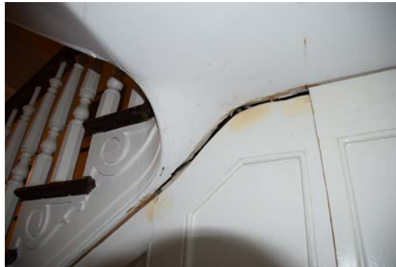
Fig. 69 [Left] Panel below stair cut to allow access to heat pump [BBB, 2024]
