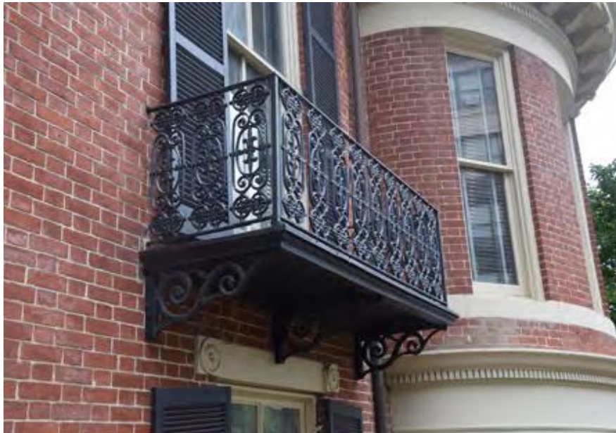
The new cast iron balconies: Photo: Beyer Linder Belle, Historic Structural Report (2021), p. 58.
