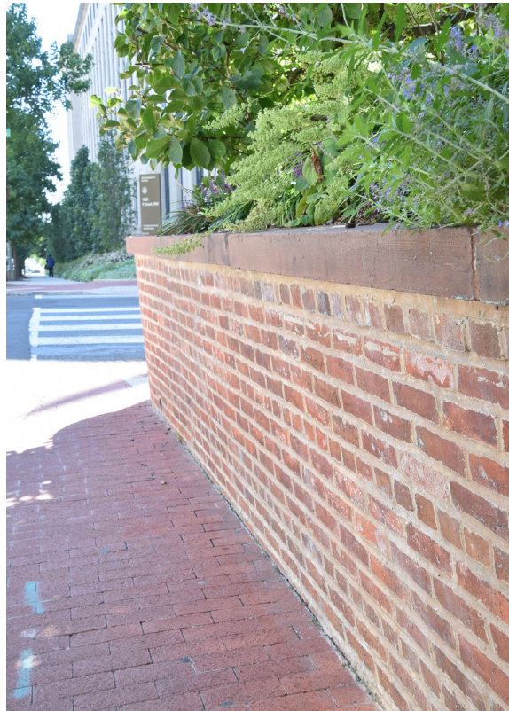
5.1 [Top Left] Southeast corner of the retaining wall showing signs of step cracking, repair, and repointing. [BBB, 2020]
