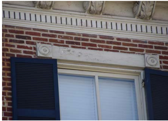
5.50 [Top Left] Checking and peeling paint at the third floor tripartite window sill and frame on the south elevation. [BBB, 2020]
