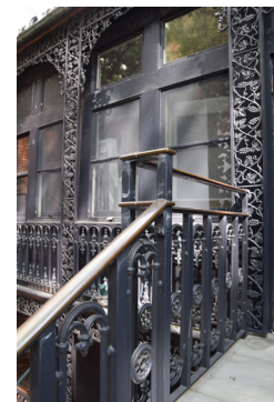
5.63 [Lower Left] Left: Metal railing and platform at southwest porch exhibits corrosion. Right: Metal steps also exhibit corrosion. [BBB, 2020]
