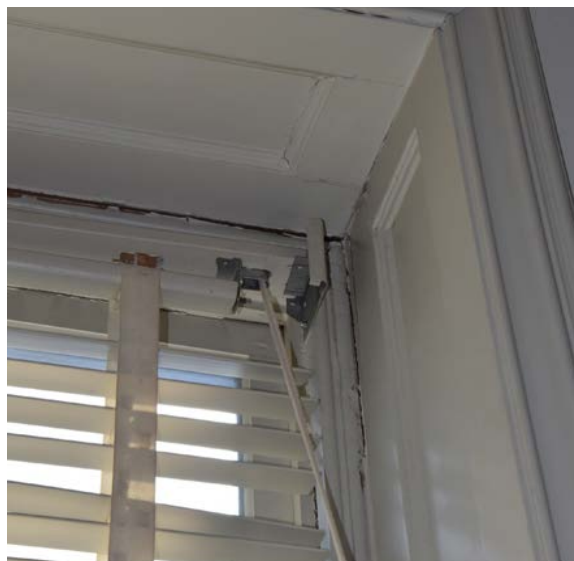
5.93 [Lower Left] Loss of profile from settling at window surround and separation of joints at window header and jamb in south central room on third floor. [BBB, 2020]
