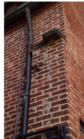
5.33 [Center Left] Previous southwest downspout showing displacement from the gutter at the overhanging cornice causing deterioration and biological growth to the masonry below. This downspout was replaced in 2021. [BBB, 2020]
