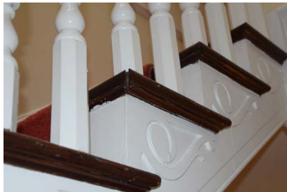
5.84 [Lower Right] Separation of joints at Main Stair nosings. [BBB, 2020]
