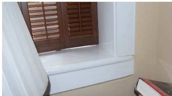
5.92 [Center Right] Loss of profile at window stool in Library on the first floor. [BBB, 2020]
