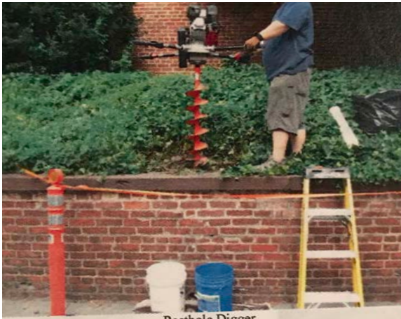
2.95 [Left] 2007 work to place additional weeping holes at the retaining wall. [DACOR Bacon House]
