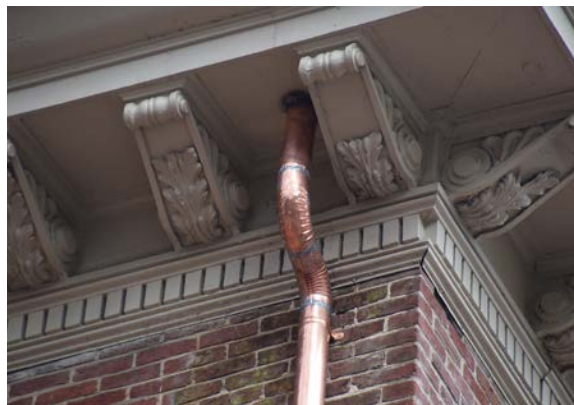
3.1 [Top] New copper downspout at the southwest corner of the House. [BBB, 2021]
