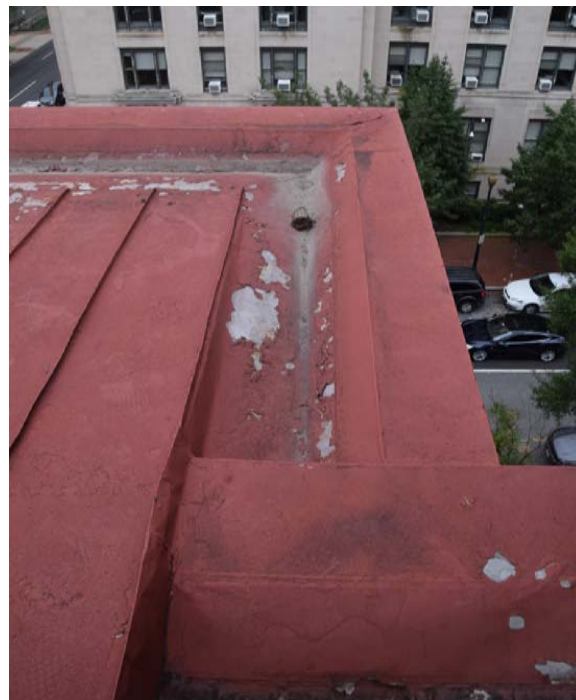
5.25 [Lower Right] Peeling paint at roof. The strainer box at the downspout is displaced. [BBB, 2020]
