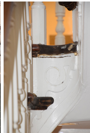
5.82 [Lower Left] Deflection at main stair from half landing to fourth floor. [BBB, 2020]
