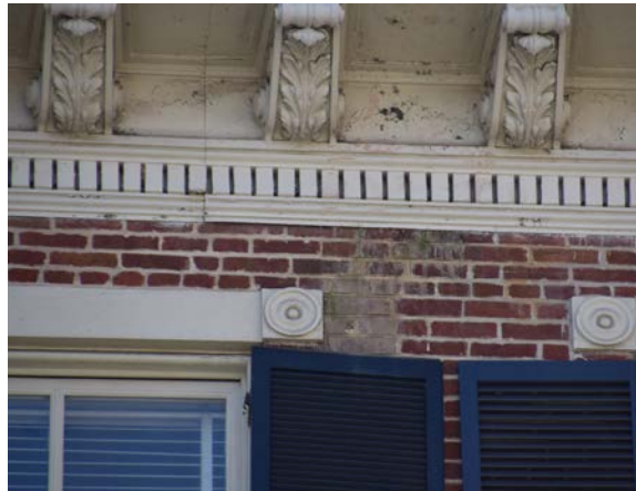
5.31 [Top Left] Peeling paint and iron staining at the galvanized sheet metal cornice, [BBB, 2020]
