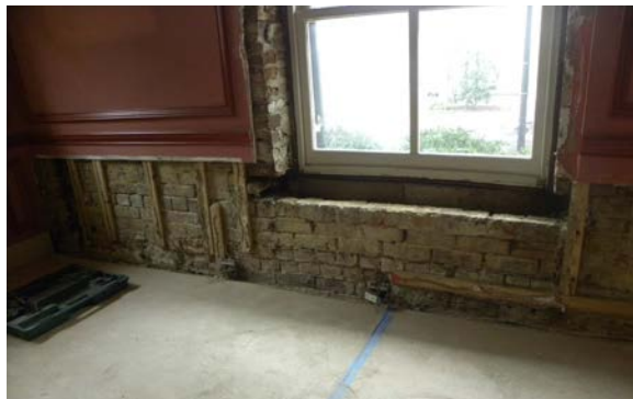
2.99 2012 photo of work following termite damage in the Ladies' Lounge. [DACOR Bacon House]
