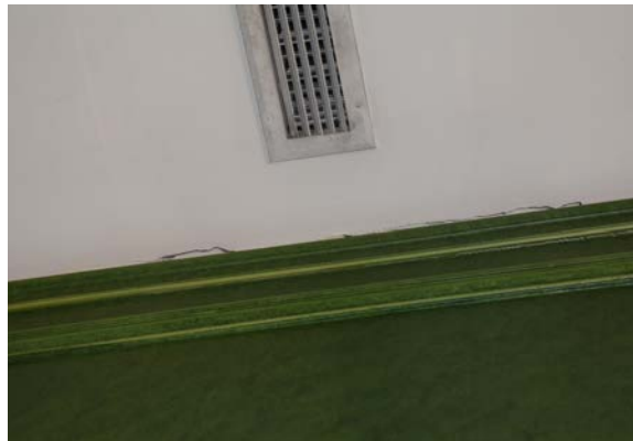
5.74 [Lower Right] Cracking at ceiling in Grand Stair on second floor. [BBB, 2020]
