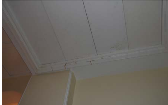
5.72 [Lower Left] Peeling paint and staining from water damage at ceiling of semi-elliptical bay within the Grand Stair Hall. [BBB, 2020]
