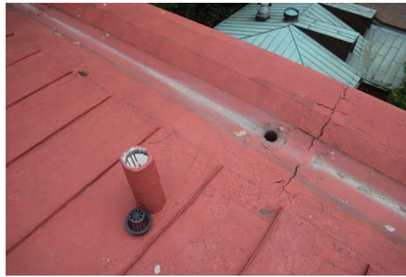
5.21 [Top Left] Northwest corner of the House roof, looking northwest. Standing seams have been flattened. [BBB, 2020]
