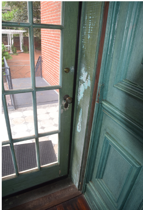
5.89 [Top Left] Worn finish and brown painted molding at the main entrance door. Door also features a bulge below the existing lock where old hardware was likely located. [BBB, 2020]
