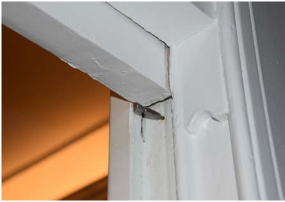
5.95 [Top Left] Metal pin installed at window frame between Dining Room and Gallery. [BBB, 2020]
