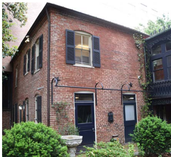
5.46 [Right] South elevation of the Carriage House showing areas of cement mortar. The brick has various finishes resulting in a patchwork appearance. [BBB, 2020]
