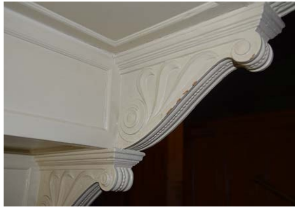
5.80 [Top Left] Staining and missing paint at Grand Stair. [BBB, 2020]
