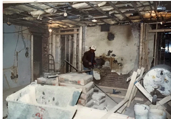
2.24 [Top Left] Circa 1980 photo of the first floor (English basement) kitchen, looking south, which is the likely location of the original Ringgold kitchen. The stove on the right is against the original fireplace and a hole in the wall above the stove indicate where an older stove pipe was likely located. [HABS Library of Congress]
