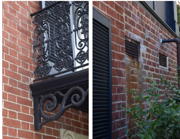
5.44 [Right] Left: Cracking at brick where cast iron balcony is attached on the south elevation. Right: Iron staining below the corroding grille at the masonry below the Gallery/north porch. [BBB, 2020]
