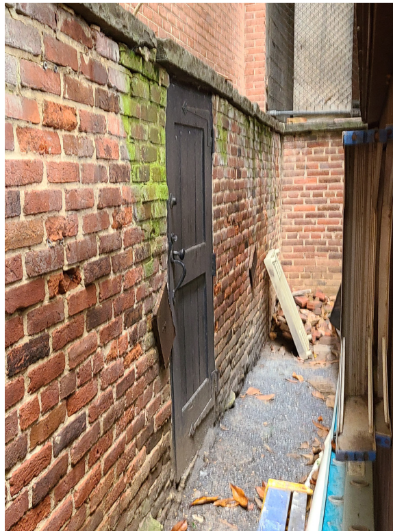
3.93 [Left] Portion of the south Garden wall showing significant bowing and structural damage. [BBB]
