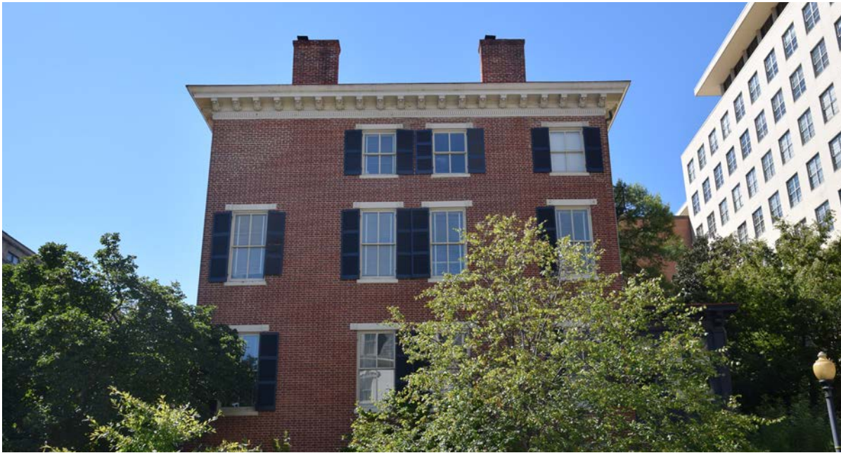
5.52 [Center] Windows on the east elevation. Several window shutters are missing or broken. The center window at the fourth floor has shutters with three panels as opposed to two panels. [BBB, 2020]
