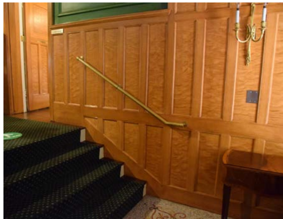
2.6 [Right] ADA-compliant handrail at the front vestibule. [BBB, 2020]
